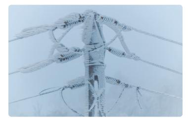
High winds may cause ice laden lines to gallop, and if the wind is significant, the galloping lines may collide causing faults, downed lines, possible equipment damage and sustained power outages.
